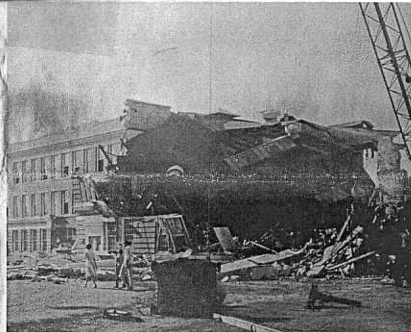
THERE SHE GOES said the crowd of onlookers and workmen alike when the south gymnasium wall collapsed in a pile of bricks after pounding and pushing by a huge four-in-one cat and the steel breaking ball. The ball, left foreground is almost as big as the little boy in flight. In the background at left of center is the high school entrance where workmen recovered the cornerstone laid by Monroe Masons in 1910.--Monitor Photo
